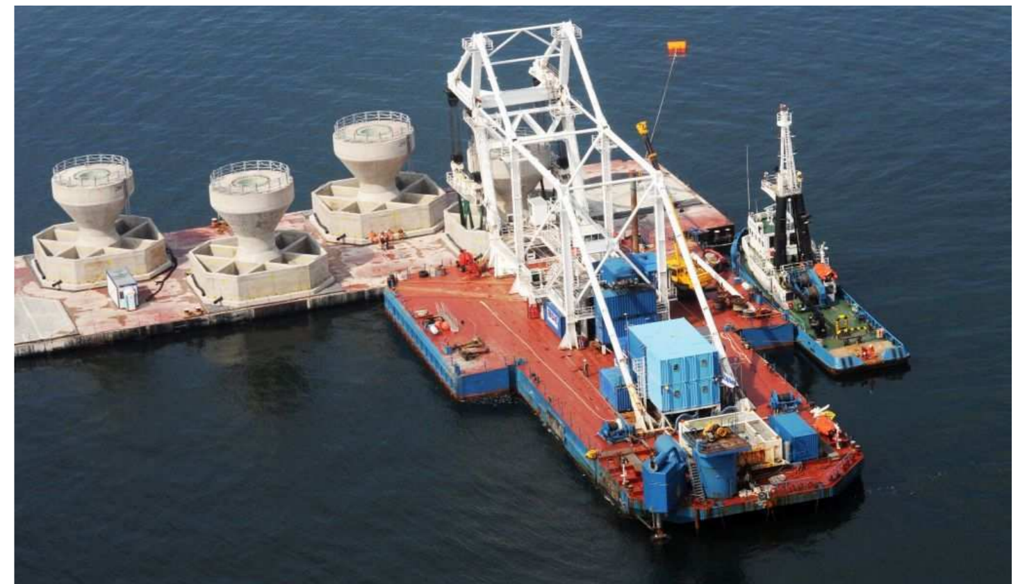
Placing of foundations
