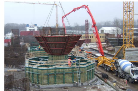
Casting of foundation structures on barge
