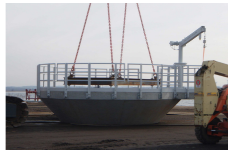
Concrete work platform
