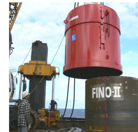
Pile driving with hydraulic hammer
