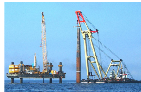
Delivery of monopile from the floating crane "ENAK"
