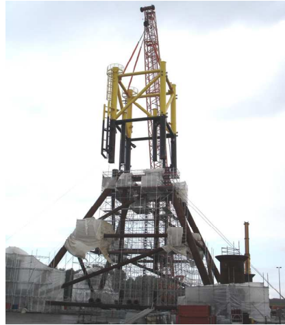
Jacket construction at quayside
